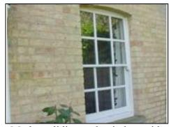
Modern sliding sash window with double glazing
