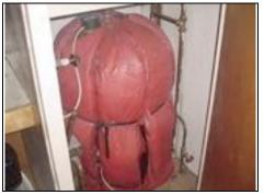
Older style cylinder with loose insulation jacket
