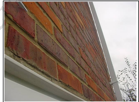
Movement to brickwork to rear French doors
