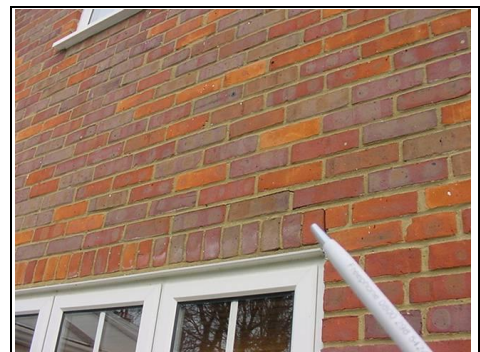
Cracking above window
