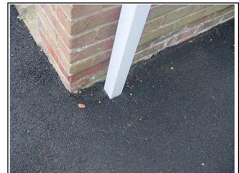
Downpipe directly into ground
