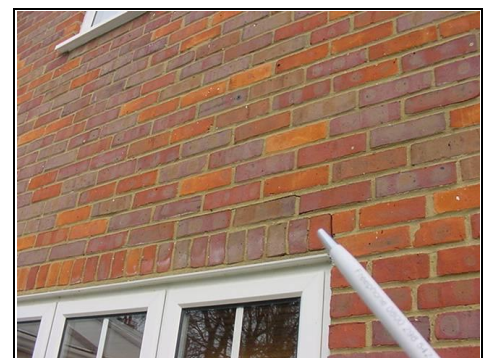
Cracking to brickwork around windows
