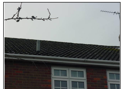
Soil and vent pipe
