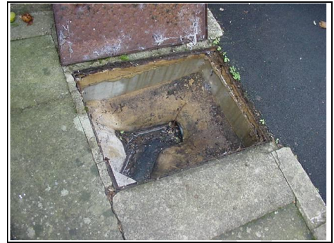
Blocked manhole
