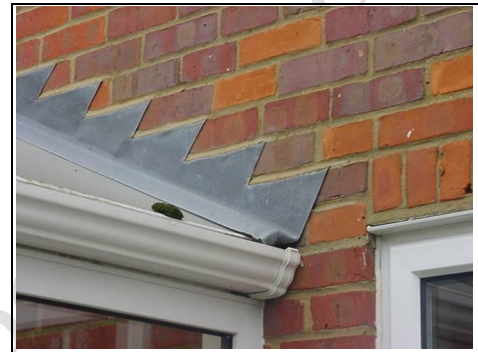
Lead flashing where conservatory meets main building
