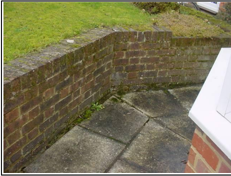
Retaining wall needs weep holes
