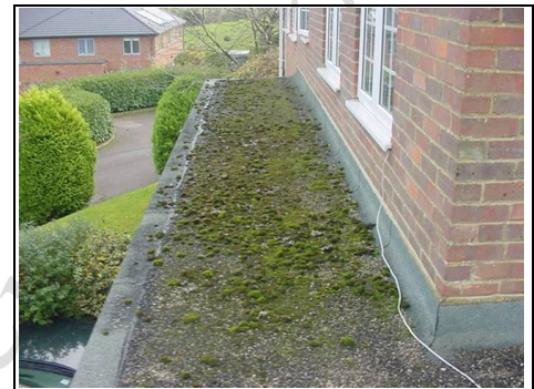
Moss on flat front roof
