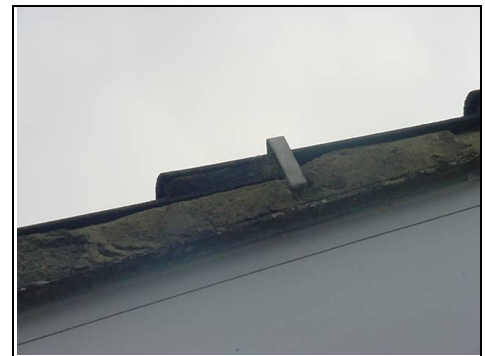
Clip to tile at edge of roof
