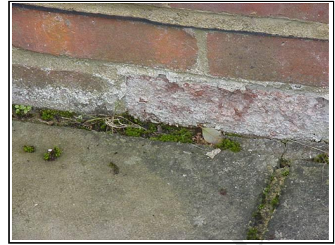
Damage to bricks due to being on a sloping site
