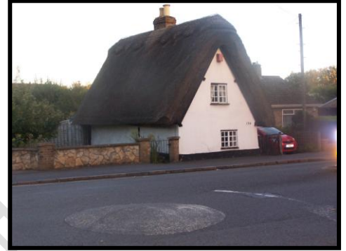
Original crux frame building – literally two trees lent against each other, the timber frame is hidden by the render
