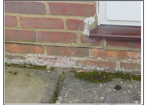
Damage to brickwork due to being on a sloping site
