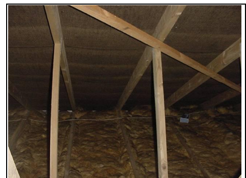
Wind brace within roof – diagonal timber
