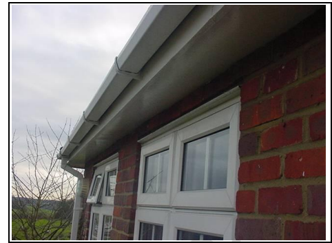
Window with no trickle vent
