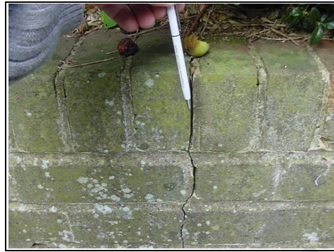
Retaining wall cracking
