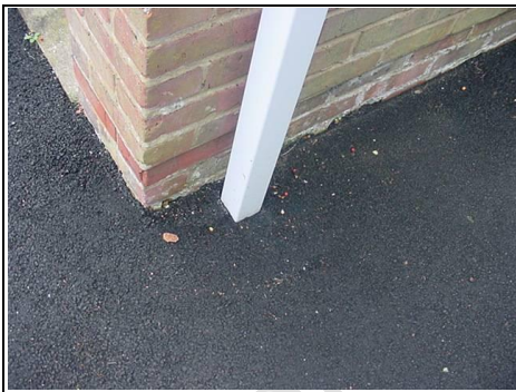
Downpipe going directing into the ground without a gulley
