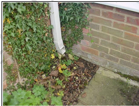
Downpipe from conservatory roof discharging onto ground
