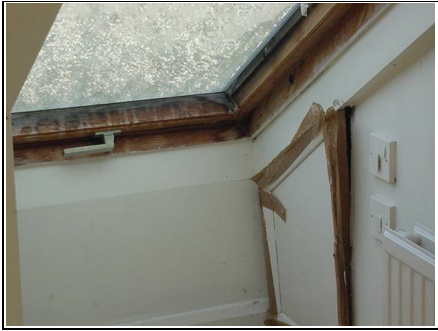
Roof window leaking
