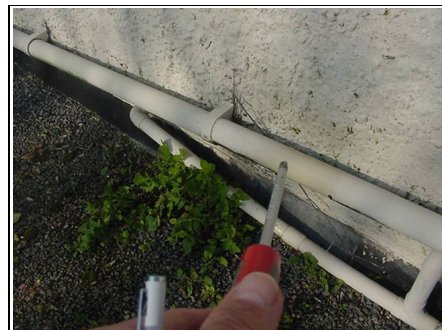
Leaking overflow pipes with grass growing at bottom
