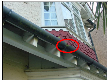
Broken gutter
