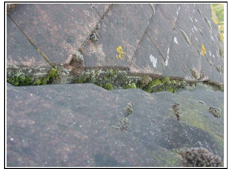
Valley gutter blocked with lots of moss
