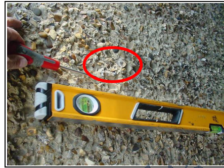
Vertical crack to render on right hand side
