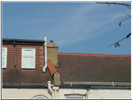
Soil and vent pipe
