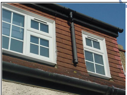
Loose downpipe to rear
