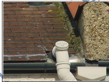
Soil and vent pipe travelling down through house
