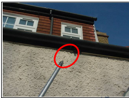
Hairline cracking in render
