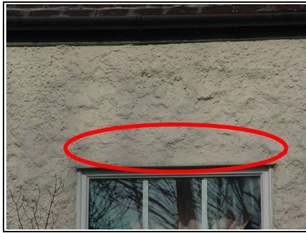
Repairs to the rough cast render above window on rear
