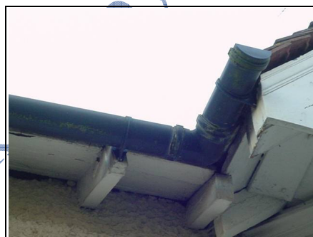
Leaking gutter
