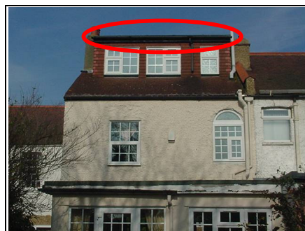
High level flat roof to the dormer
