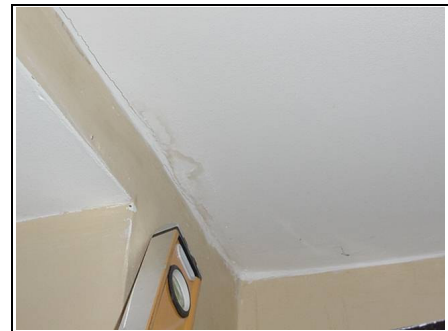
Dampness in ceiling below bathroom
