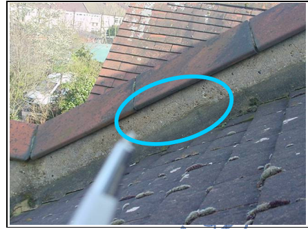
Cracking and movement to parapet wall and moss on roof tiles
