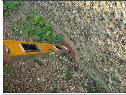
Air brick acting as a gutter to right hand side of property
