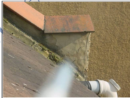
Cracking to rear of left hand parapet wall
