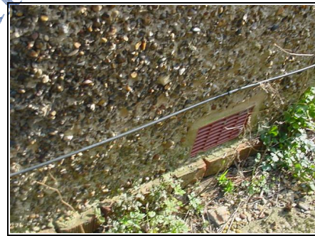
Air brick acting as a gutter to side of property
