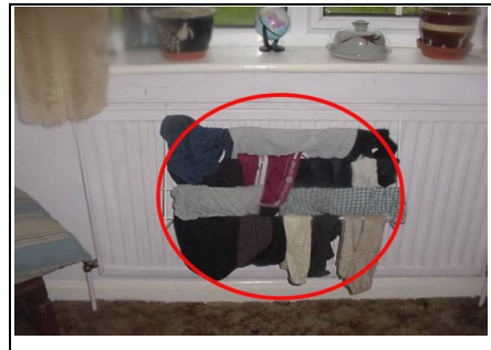
Washing drying on radiators creates moisture
