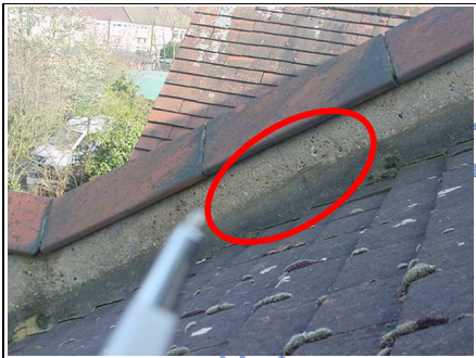
Pen indicates crack and deterioration in left hand side high level parapet wall
