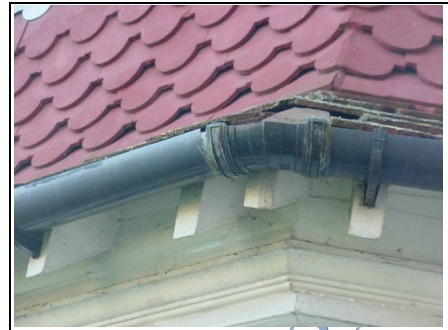
Poorly jointed guttering
