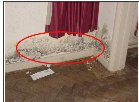
Mould caused by cold bridging
