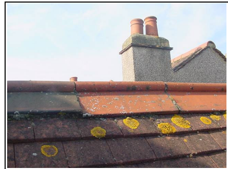
Ridge tiles have been replaced
