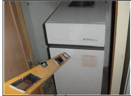
Floor mounted Kingfisher boiler
