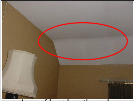
Area of heat loss through a sloping ceiling
