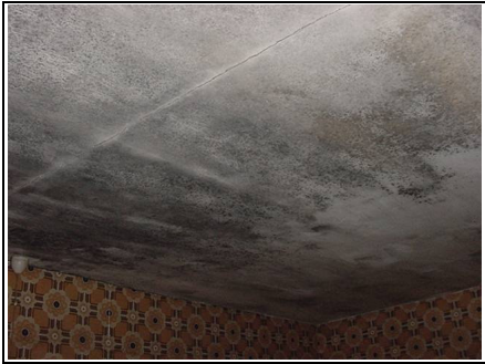
Ceiling covered in black mould
