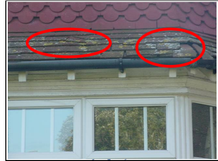
Slipped/broken tiles over bay window
