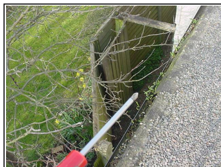
Flat roof gutters full of plants that needs clearing
