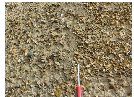
Different sorts of render, with modern pebbledash to the right hand side
