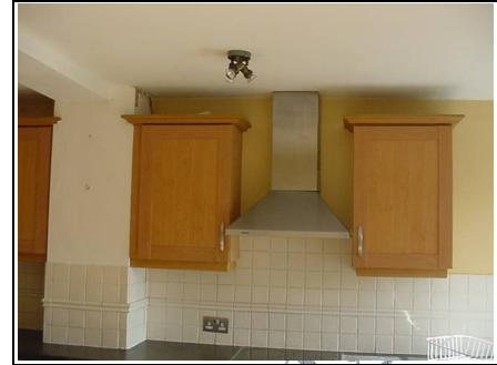
This filter in the kitchen is not an extractor
