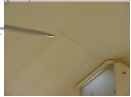
Hairline cracking in top room ceiling
