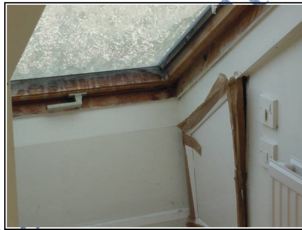
Dampness coming through roof windows causing deterioration to window frames
