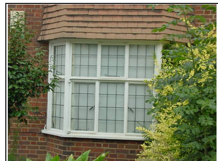
Metal Crittall can suffer from cold bridging
