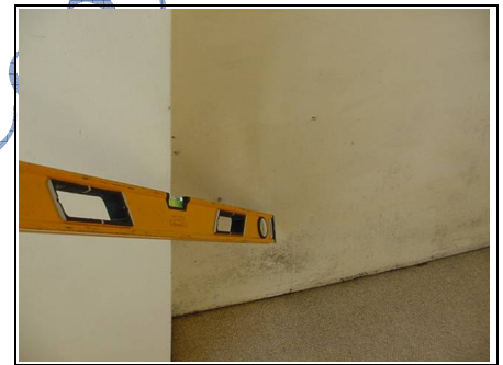
Black mould on top floor
