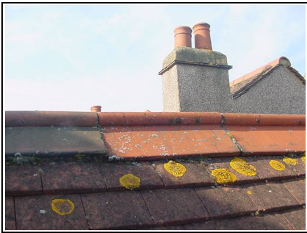
Ridge tiles have been replaced
