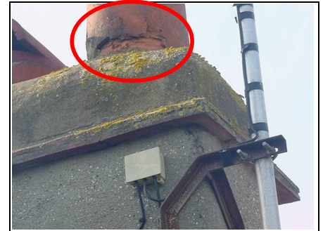
Spalling to base of chimney pot
