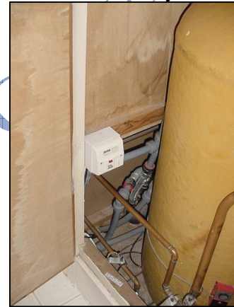
Plastic pipes next to water cylinder that may leak
