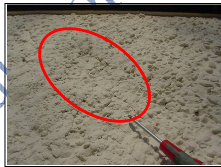
Hairline cracking
