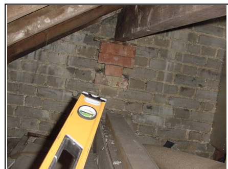
Brick fire wall to left hand side
