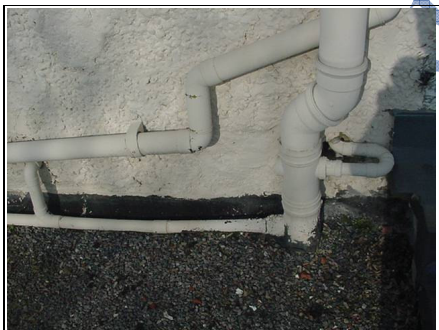
Awkward soil and vent pipe
