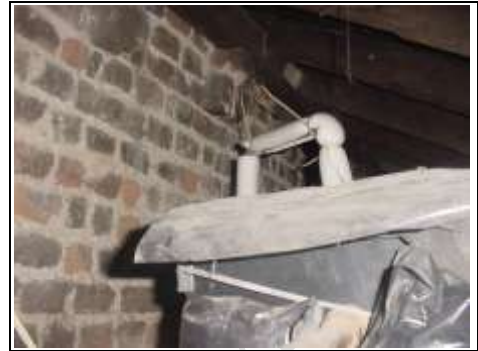
Top up tank for the central heating
