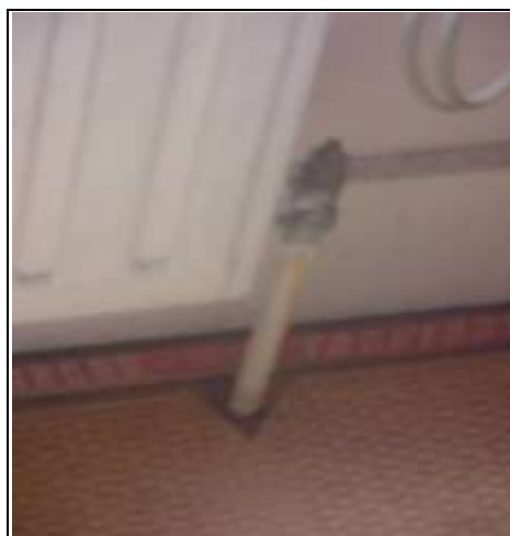
Leaking radiator pipe
