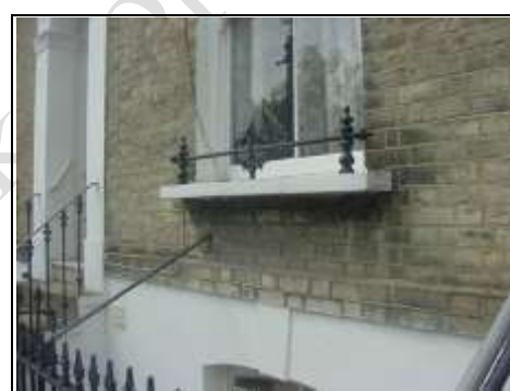
Flemish bond brickwork
