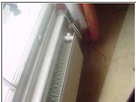
Leaking radiator on the upper ground floor causing possible dampness to the lower ground floor
