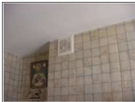
Vent to chimney breast in kitchen
