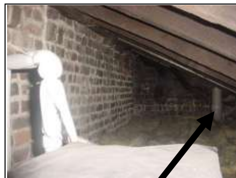
Internal soil and vent pipe in the right side roof
