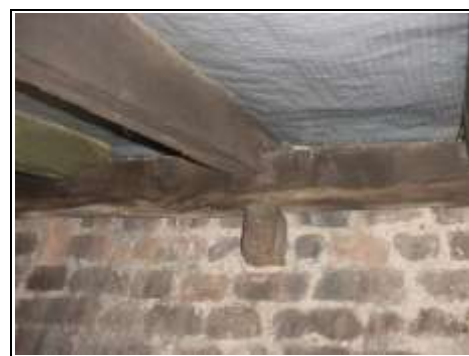
Dampness visible to timbers on the left hand side of the London Butterfly roof
