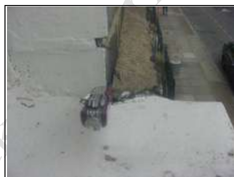
Brick work stringer with a cement fillet. The knife in the gap shows how dampness can get behind it
