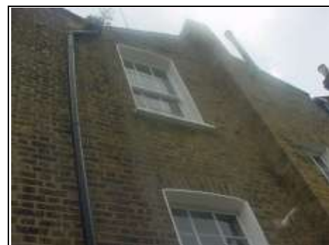
Pattern staining caused by the hopper head over flowing
