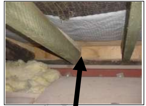
Staining to the timber of the valley gutter. This could be causing dampness in the bedrooms at first floor level
