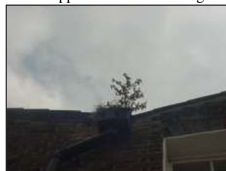
Plant growing in hopper head to the rear. Bigger hopper heads are needed.
