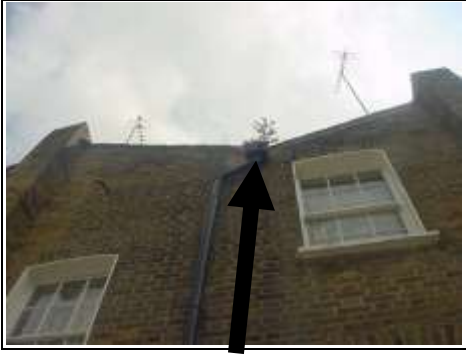
Plant growing in the hopper head to the rear of the property. This could be allowing dampness in at first floor level
