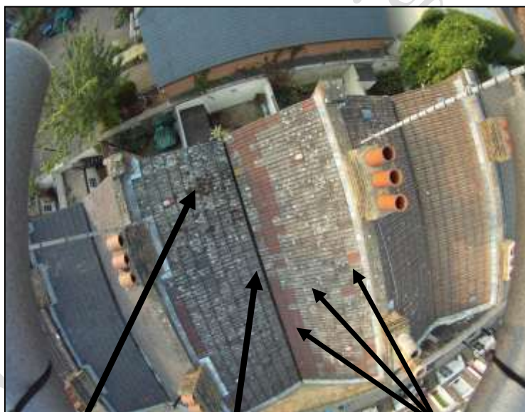
Lichens Narrow Valley Gutter Different coloured tiles
