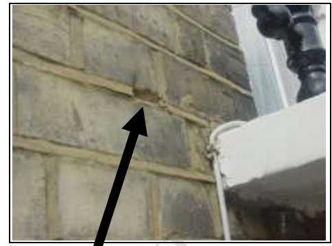
Cement mortar falling out to the front of the property. If you recall we took a bit out.
