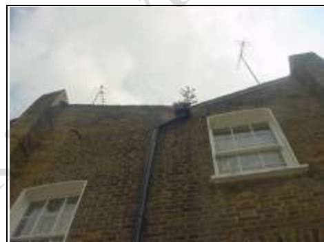
Hopper head to the rear of the London butterfly roof
