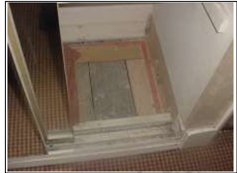
New floorboards in the cupboard may relate to central heating being put in or it may relate to woodworm problems
