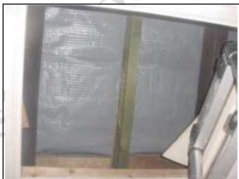
Torn protective underlayer - right hand roof.
