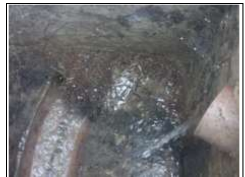
Manhole (middle right)
