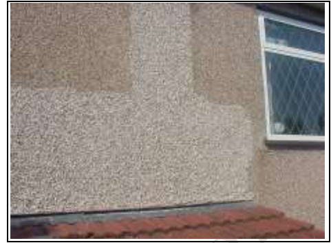
Chimney has been removed to the rear of the property
