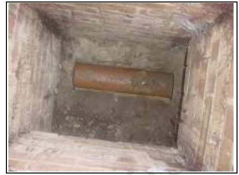
Manhole (front right)
