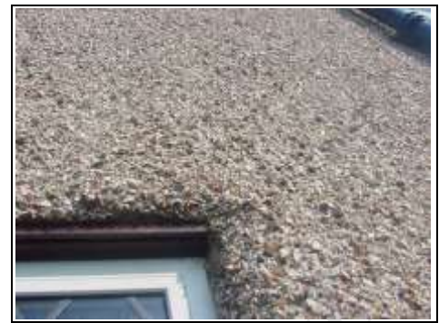
No drip detail over the window
