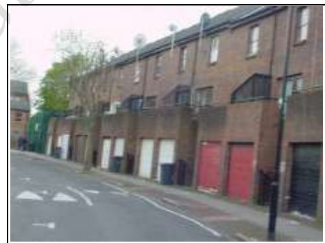
1960's properties built with concrete lintels that can cause Cold Bridging
