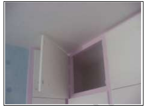
Built in cupboards
