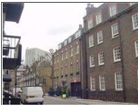
Older style London converted flats with property problems such as Condensation and Cold Bridging
