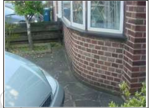
Brick work detail to front bay
