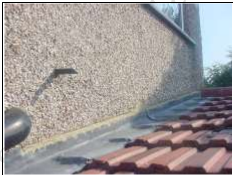
Flashing where the extension meets the main building
