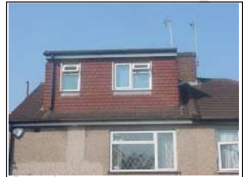
Rear of loft conversion
