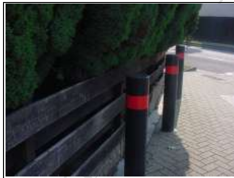
Posts in front of garden fence
