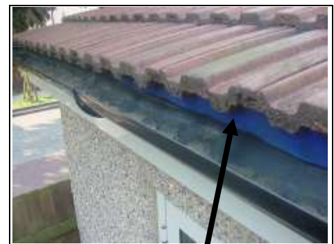
Underlayer visible on pitched roof
