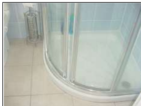
Tiled floor on timber in en-suite shower room
