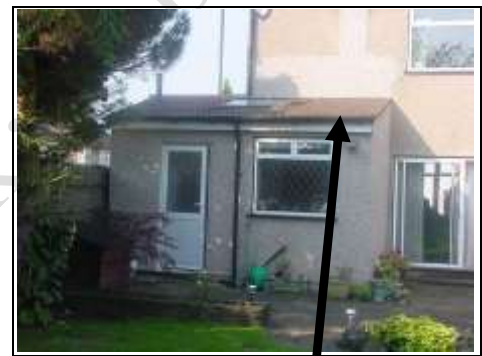
Shallow pitched roof to kitchen extension
