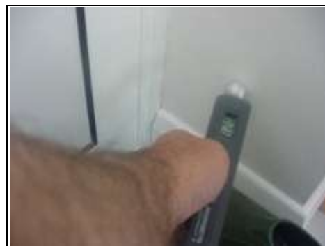
Testing for rising damp
