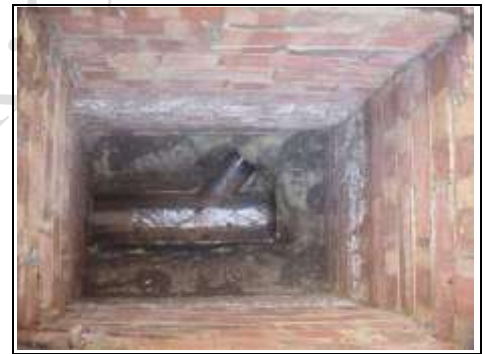
Manhole (middle right)
