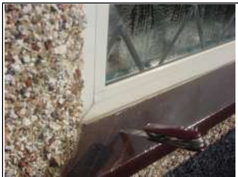
Testing the timber windows with a knife
