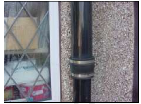
Combination of cast iron and plastic soil and vent pipe
