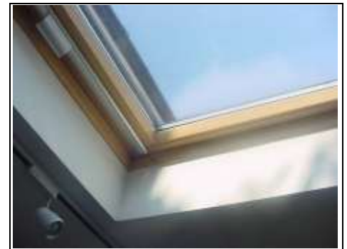
Roof window from within kitchen
