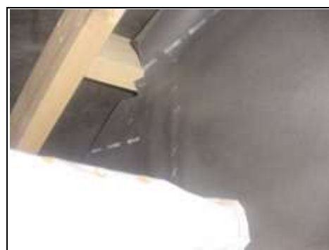
Limited view of roof timbers
