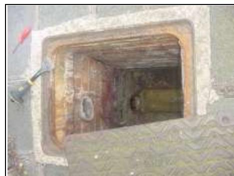
Manhole (front left)
