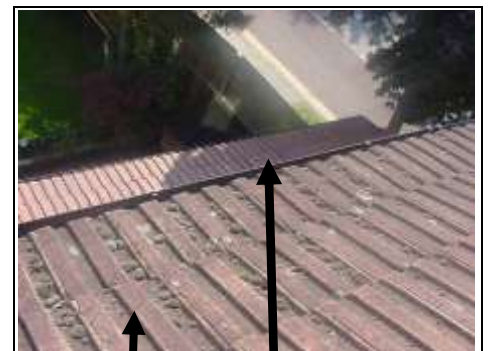
Main roof. Shallow pitch roof.
