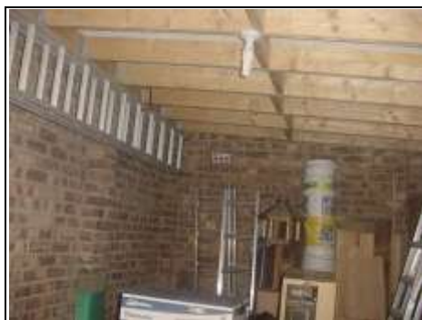
Inside the garage
