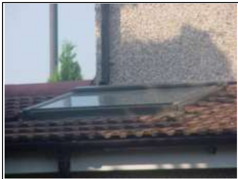
Roof window to the rear extension
