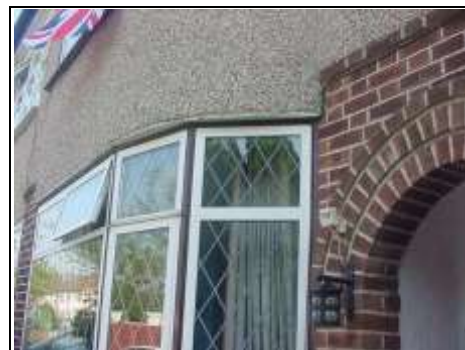
Timber double glazed windows
