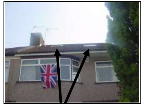
Roof windows (front)
