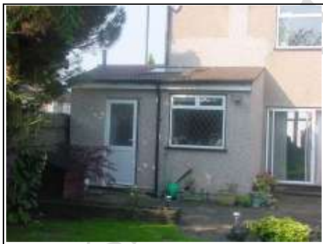
Shallow pitched roof to kitchen extension
