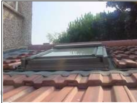
Roof window to rear extension roof
