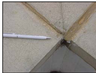
Mastic used to seal joints
