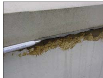
Mastic used to seal joints
