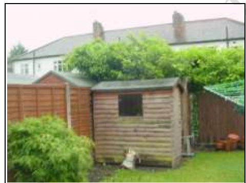
Shed to the rear
