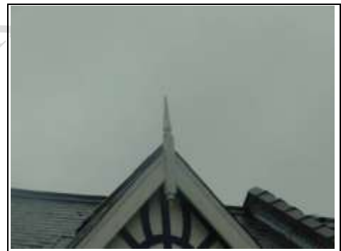
Fascias soffits and bargeboard
