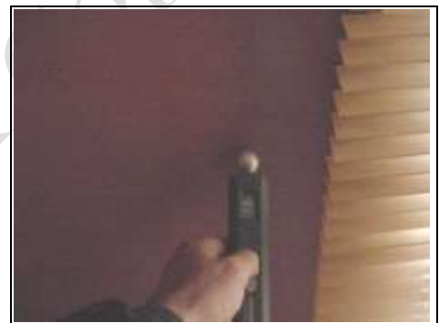
Testing for lateral dampness
