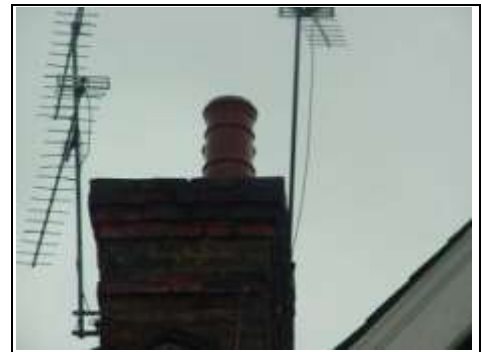
Close up of chimney One
