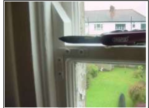
Window held together by metal straps
