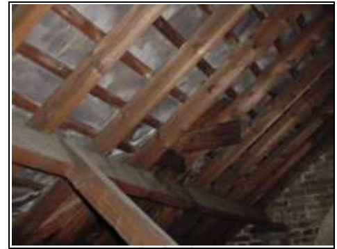
General view of inside of main roof
