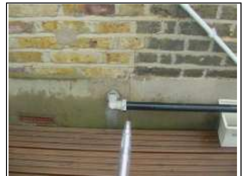
Different brickwork to rear
