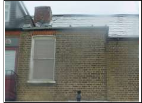
Flat roof to rear
