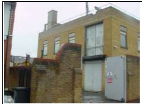
British Telecommunications Telephone Exchange building nearby
