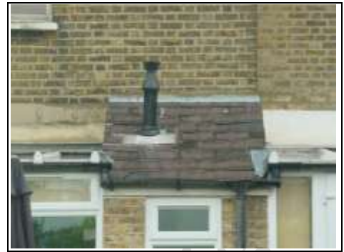
Rear low level slate roof
