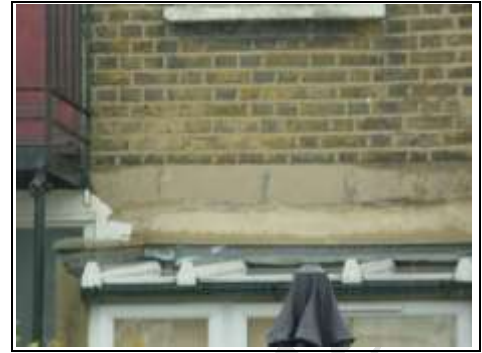
Polycarbonate roof over kitchen
