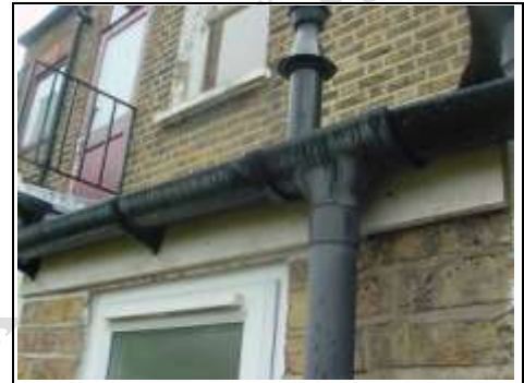
Gutter and downpipe
