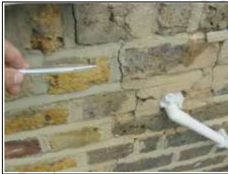
Cement mortar re-pointing
