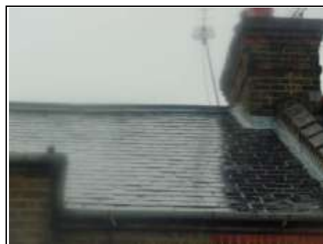
Rear roof undulates
