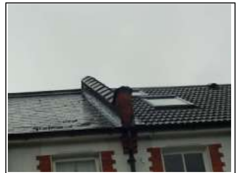
Next door's loft conversion with concrete tile to right hand side and your roof to the left hand side
