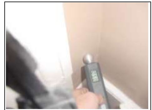
Testing for rising damp
