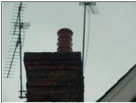
Front left hand chimney
