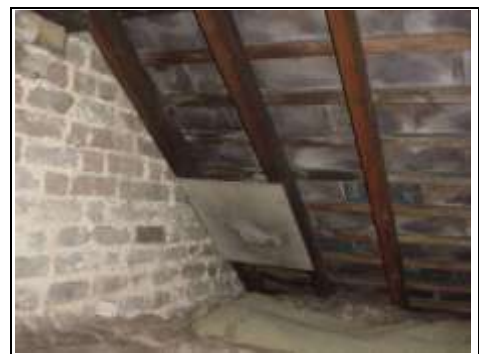
Underside of roof showing slates and piece of asbestos
