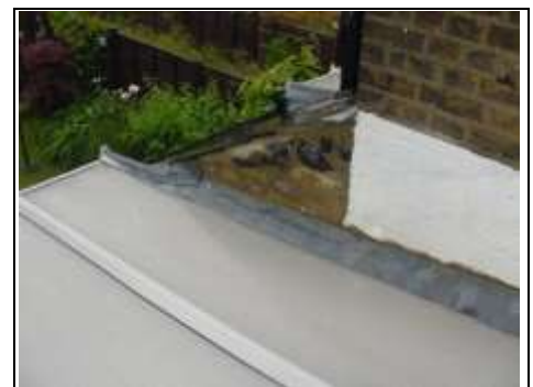
Polycarbonate roof over kitchen
