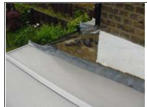
Polycarbonate roof over kitchen area 19
