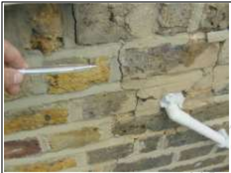
Cement mortar re-pointing
