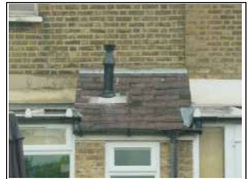
Low level slate roof
