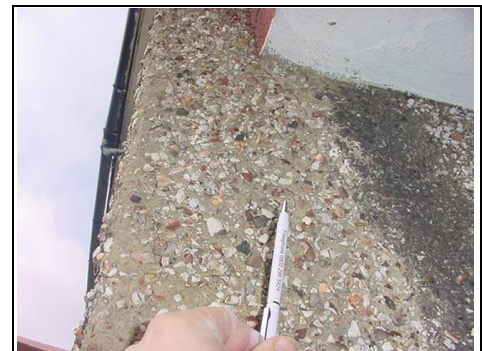
Vertical hairline cracking
