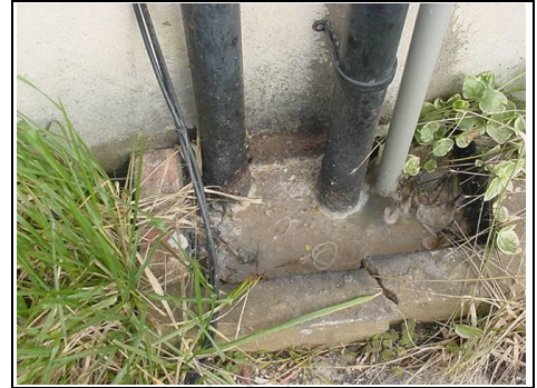
Blocked gulleys
