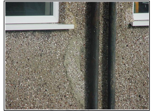
Peashingle badly repaired where there is a crack beneath that has been hidden
