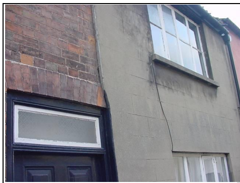
Cement Stucco render – you can tell it is cement from the colour and you can also see the pattern staining below the window.
