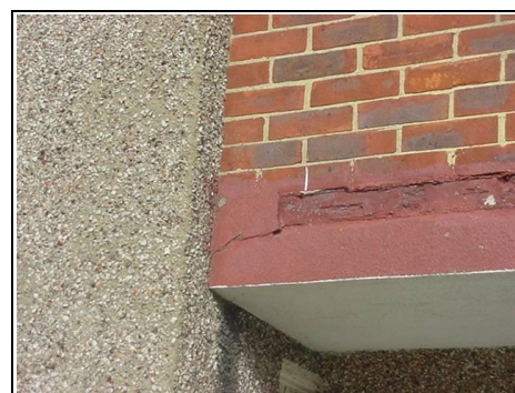
Deterioration to concrete frame
