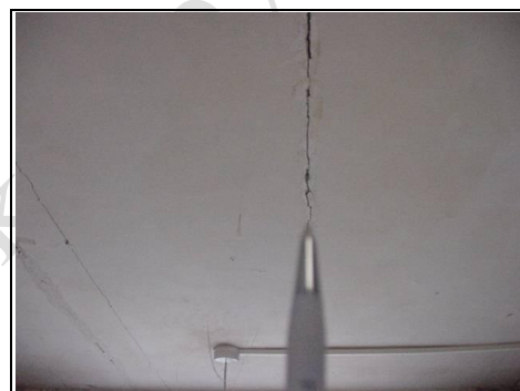
Cracking to ceiling
