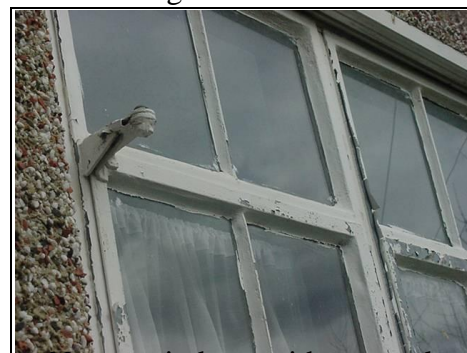
Newer windows with external hinges
