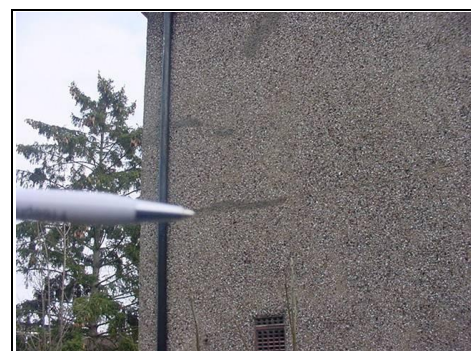
Horizontal cracking
