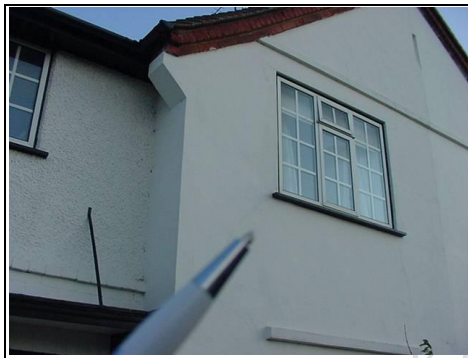
Pen indicates hairline cracking
