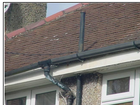
Soil and vent pipe
