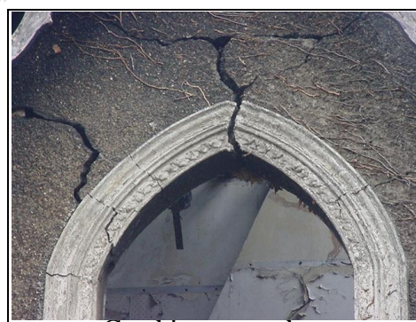
Cracking to render
