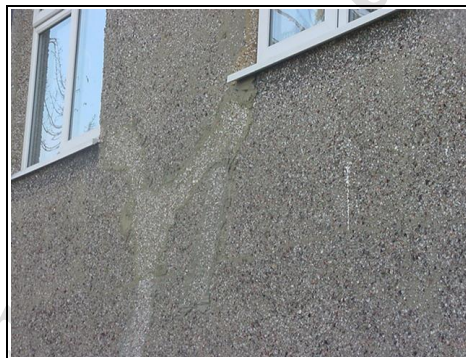
An area where Peashingle has been better repaired but still stands out where there is cracking beneath it.
