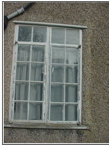
If you look closely this relatively new window has been put in place with a different texture of pebbles around the window compared with the original pebbledash.
