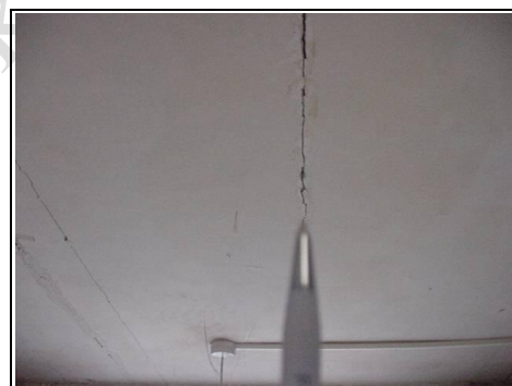
Cracking to ceiling
