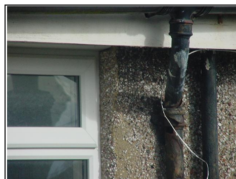
Cast iron downpipe rusted
