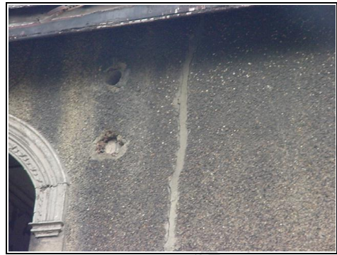
Crack brought about by expansion and contraction of the building.
