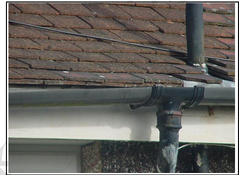
Cast iron to plastic guttering
