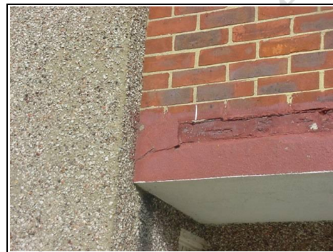
Deterioration to concrete frame
