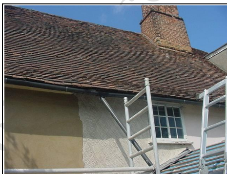
You can see what is known as the scratch coat to the right hand side which is applied before the final coat
