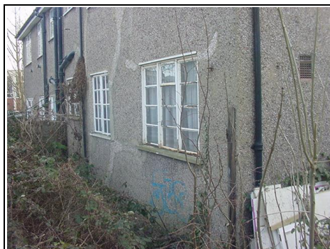
Cracking to render to rear of property
