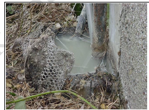
Rear drain blocked
