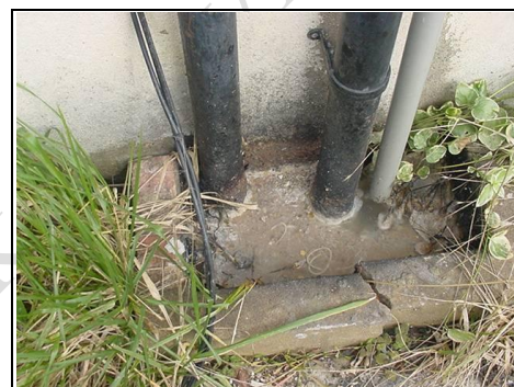
Gulleys blocked
