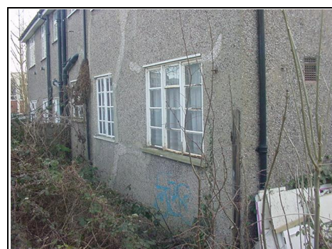
Cracks to rear of property
