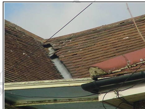
Slipped tile to hipped roof
