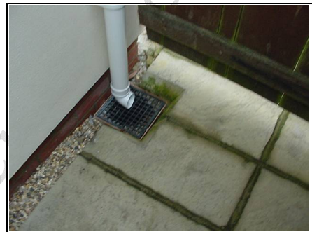
Overflowing downpipe assumed due to green moss
