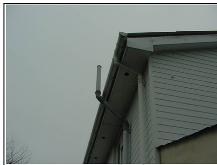
Soil and vent pipe
