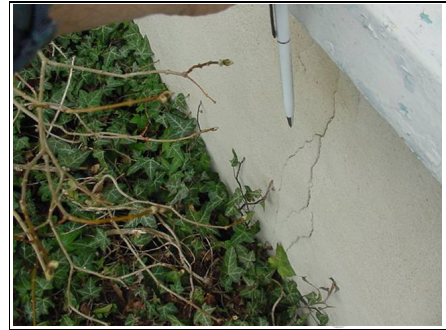
Crack to render at the rear of the property
