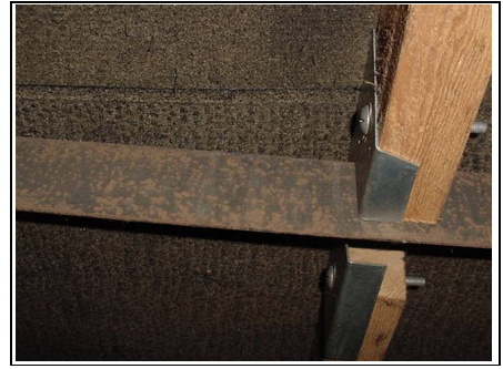
Some fixing have been replaced
