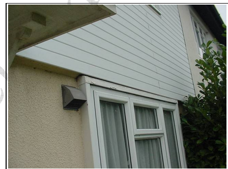
No trickle vents to window
