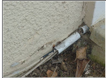
Electrics should be underground
