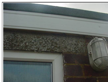
A close up view of the concrete lintel
