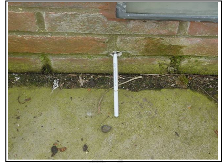
Weep holes to rear wall
