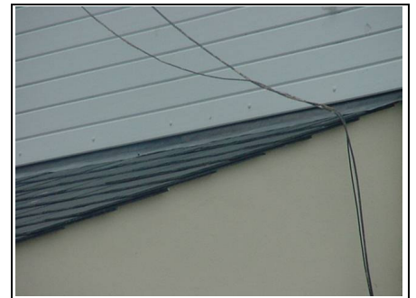
Flashing to top of the roof
