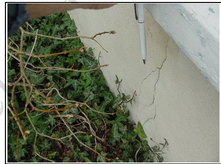
Cracking to render at rear
