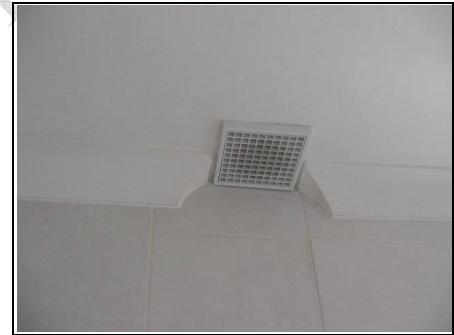
Small extract fan in bathroom
