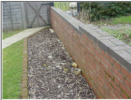
Left hand boundary wall to the front of the property would benefit from re-pointing
