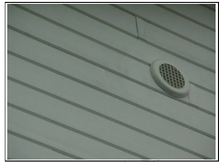
Outside vent on small extractor from bathroom
