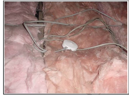
Electrics sitting on top of the insulation
