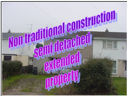
This metal framed property is in its original condition apart from the replacement roof
