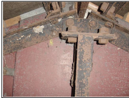
Close up showing roof bolts with more rust than we would like to see
