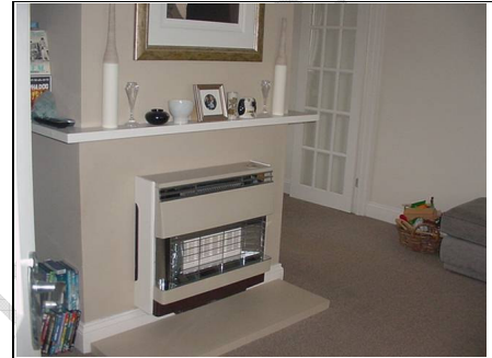
Chimney breast with Baxi Back boiler
