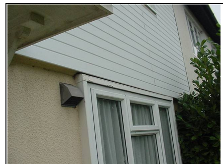
Cladding and stipple render to the front
