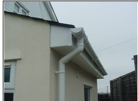
Fascias and soffits on extension without vents as it has got a breathable felt
