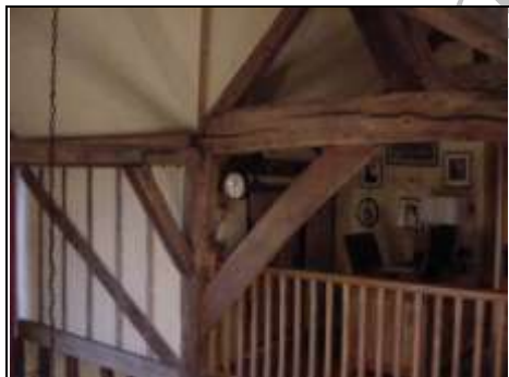
Brace between post (vertical timber) and beam (horizontal timber)
