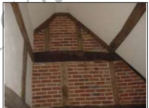
Hidden timber frame (within the walls) visible internally
