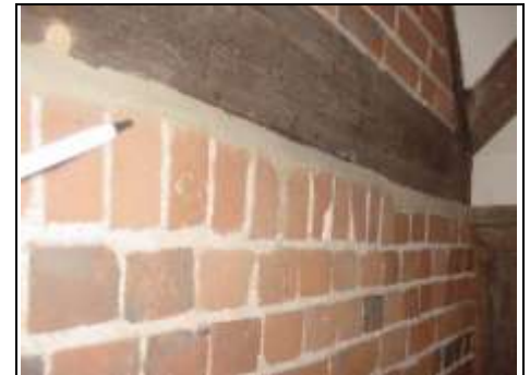
Repairs to party wall on right hand side
