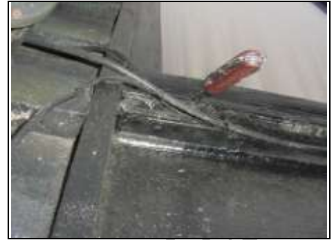
Rot in timber windows where the front door used to be
