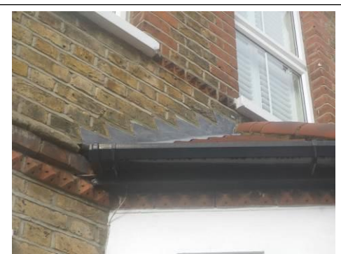
Stepped flashing and cement
