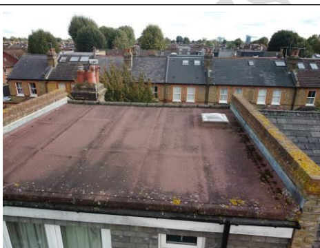
High level flat roof and parapet walls
