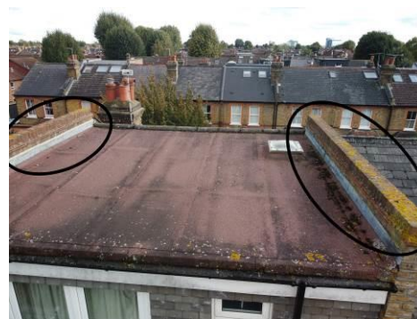
Parapet walls to rear high level flat roof
