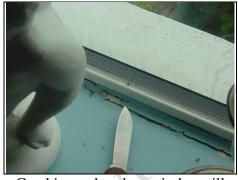
Cracking to box bay window sill on first floor rear window
