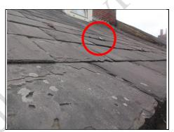
Deteriorating slates (tingle circled)
