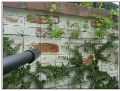
Spalling brickwork to rear garden wall
