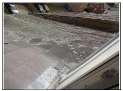
Deteriorating slates to right
