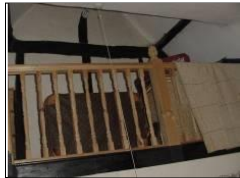
Mezzanine/roof access to right roof
