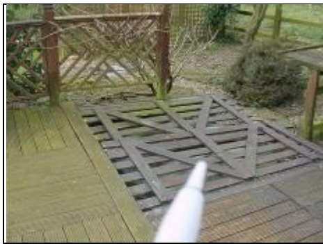
Top of septic tank
