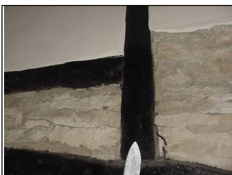
Infill panels and stonework
