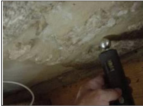
Testing for dampness in fireplace stonework
