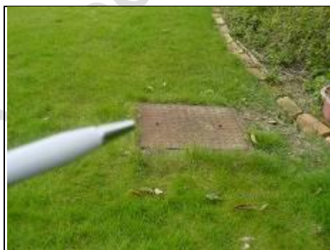
Manhole adjacent to garage
