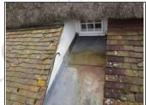
Lead valley to bathroom window
