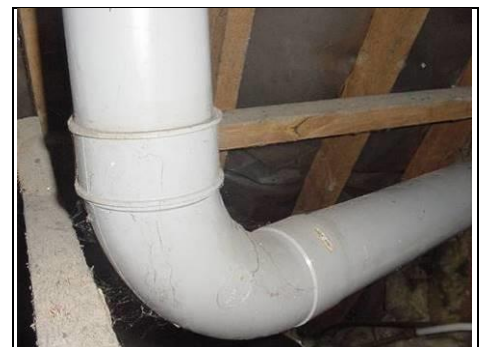
Plastic pipe within roof
