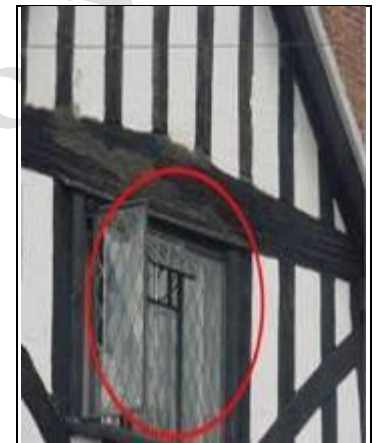
Old style diamond panel lead light in cast iron window opened to air room
