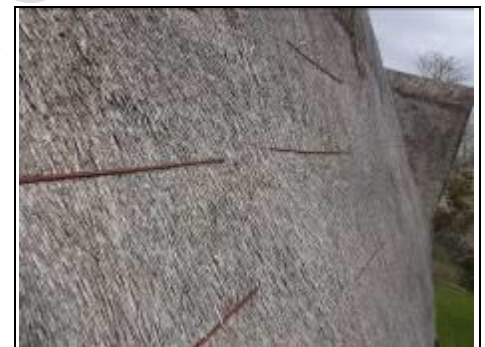
Stitch in time to thatch, rods added to hold thatch in place ~ Aerial View - 360 Photo ~
