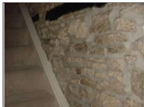
Cement repairs to stonework on side of staircase
