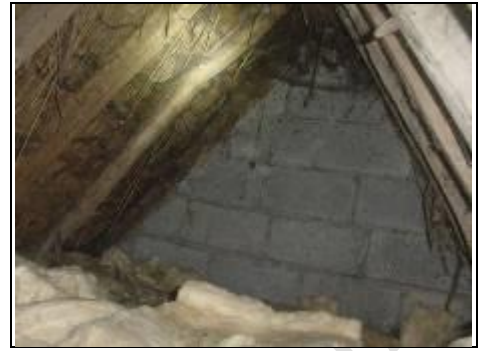
Stonework or blockwork?
