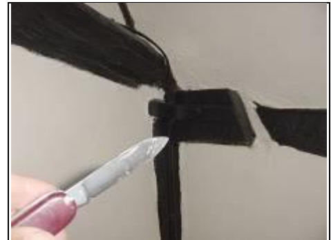
Brace added in middle wall on left side
