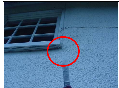
Cracking
