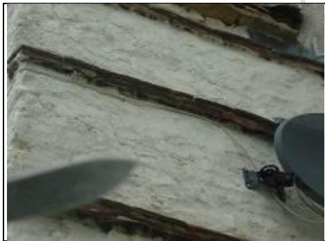
Cement repairs on stone chimney
