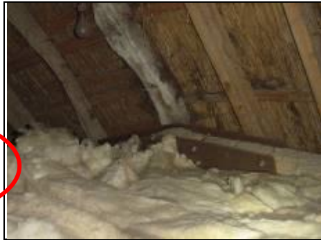
Brace at base of timber
