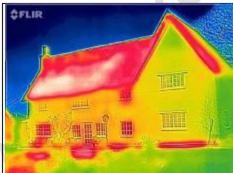
Heat coming out of floor, windows and roof to rear of property and little sign of the timber frame
