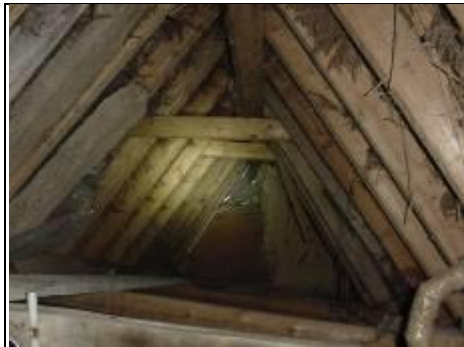
Most of timbers replaced in main part of roof
