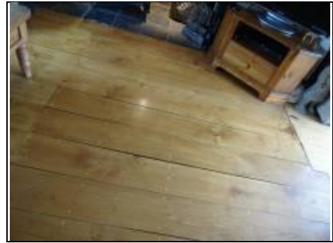
Replacement of original floorboards
