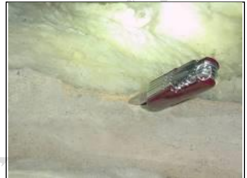
Knife going completely into timber common rafter
