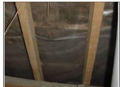
This photo shows the common rafters (the ones that form the pitch of the roof) and the dark area between is the underlayer.
