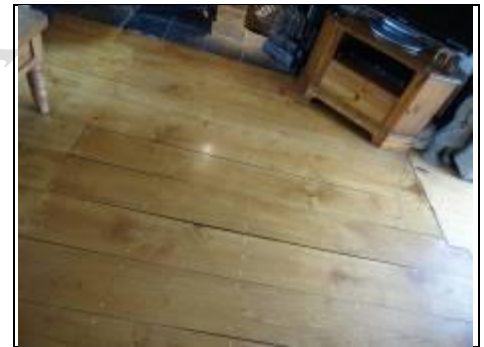
We were advised original floorboards were sanded and reshaped
