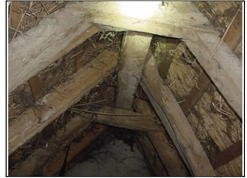
Timber to the right roof
