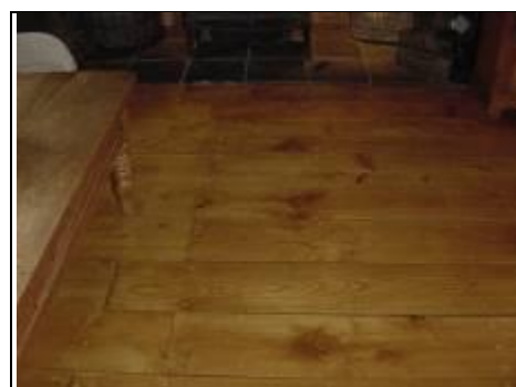
New floor made out of old flooring in main reception room
