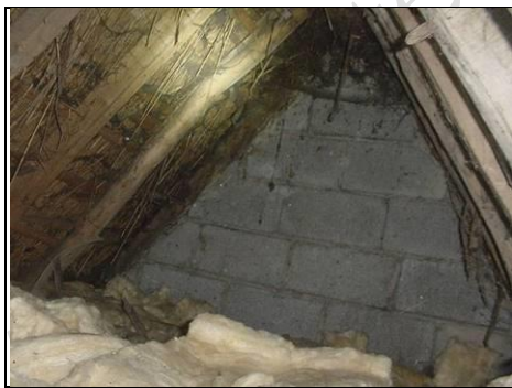
Stonework or blockwork?
