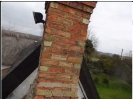
Close up of chimney
