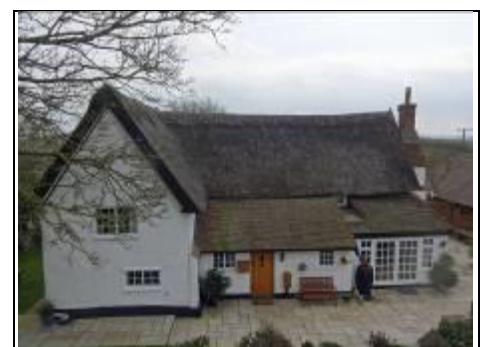
Front view of a thatched property
