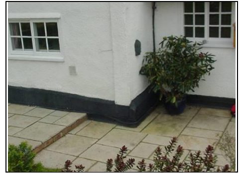
Paving around property
