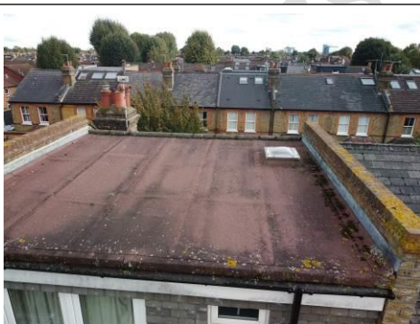
High level flat roof and parapet walls
