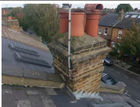
Water trap behind chimney
