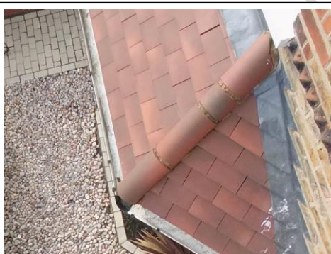
Front bay roof
