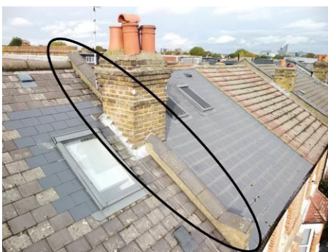
Front right parapet wall
