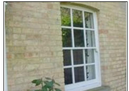
Modern sliding sash window with double glazing
