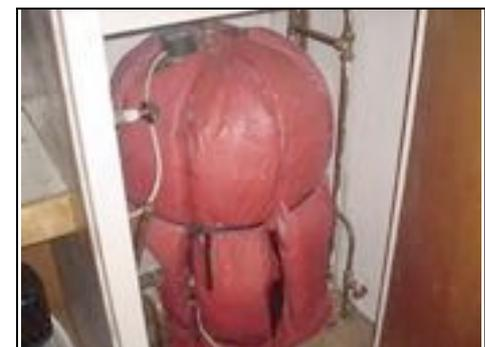
Older style cylinder with loose insulation jacket
